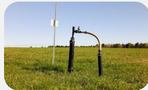
Biogas collector Intermunicipal waste management of la Lièvre.
