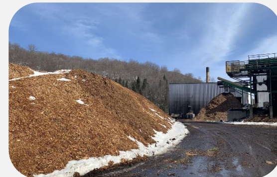
Mont Blanc site and biomass collected for dryers.
